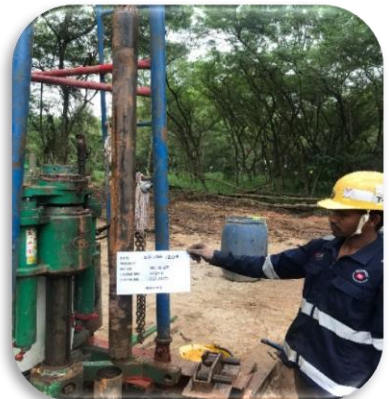
Undisturbed soil sampling: Thin-walled Tube Sample
